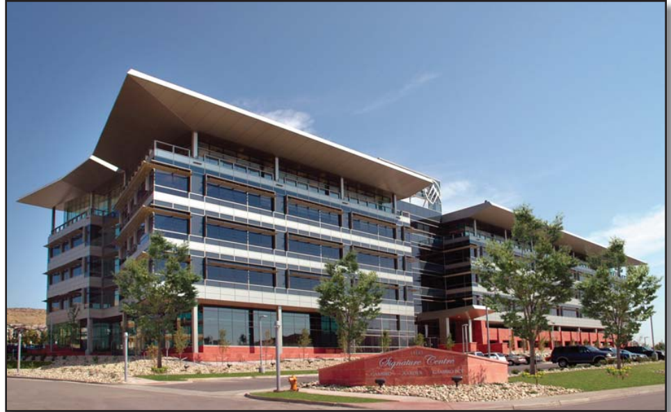
Signature Centre at Denver West is one of only 2 buildings in the world to achieve a double LEED Platinum rating by the United States Green Building Council.
